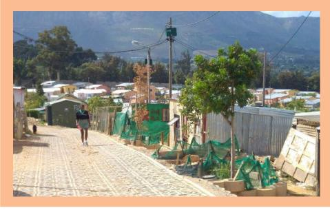
Permeable paving constructed between homes in the informal settlement of Langrug, near Franschhoek, South Africa. Surface hardening leading to poor infiltration, coupled with poor water management systems resulted in wastewater and sewage flowing through the streets. This was addressed with an integrated green and grey infrastructure approach: a combination of permeable pavements, wastewater deposit points and insertion of pipelines.
