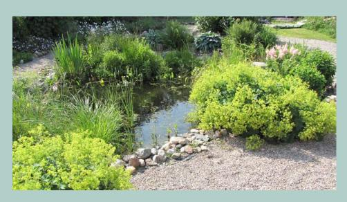
Greywater dam – a constructed wetland – where wastewater purification is based on green phytotechnology. The treatment takes place in three steps: first the sludge from the greywater is composted in a reed bed; next, the separated greywater is recycled by a pond with plants via a water ladder for oxygenation; and finally, the purified water is spread over a small gravel bed, or stone coffin, below the ground.
